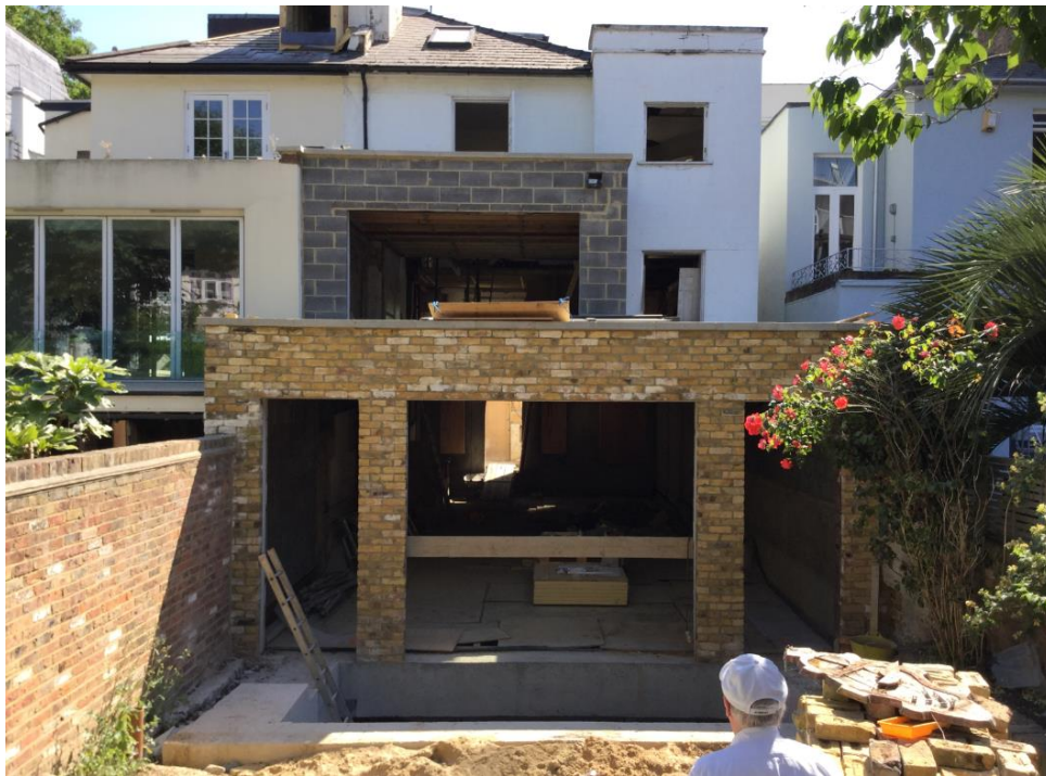
Rear of application site
